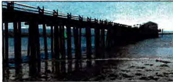
2 - PIER LOOKING SSE
