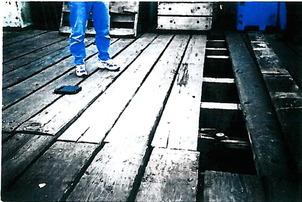
STRINGER AND PILE CAP INSPECTION PHOTOGRAPH NO. 6
