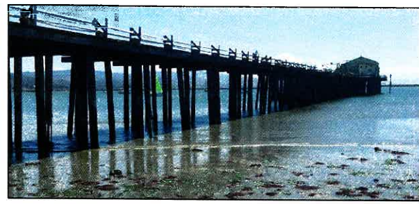
2 - PIER LOOKING SSE
