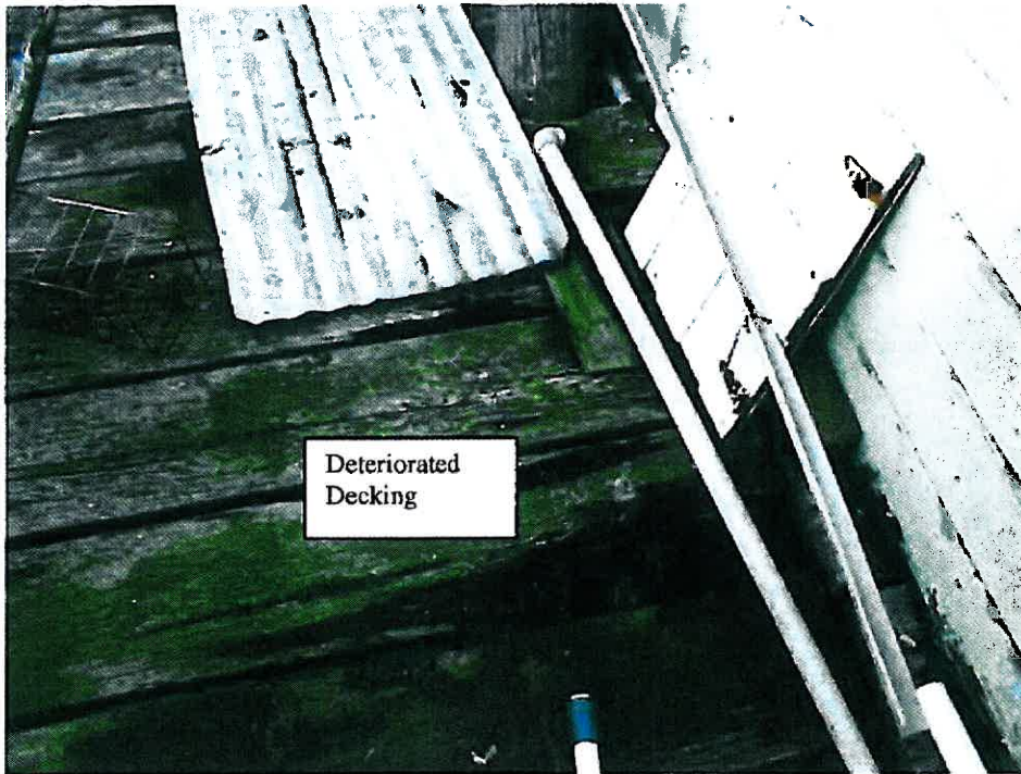
Photograph 2 – West Side of Building
