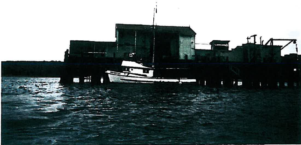
SOUTH END OF PIER LOOKING WEST SHOWING FISH HANDLING BUILDING PHOTOGRAPH NO. 2
