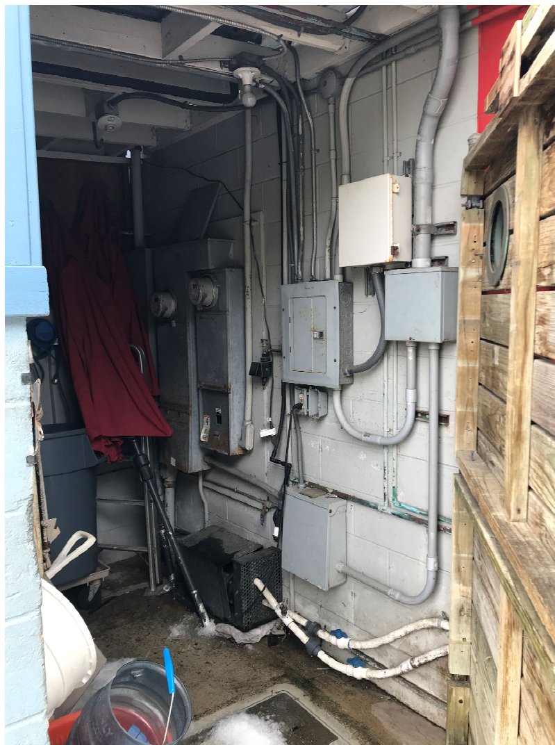
35 – View of Tenant Row Building electrical panels and storage area
