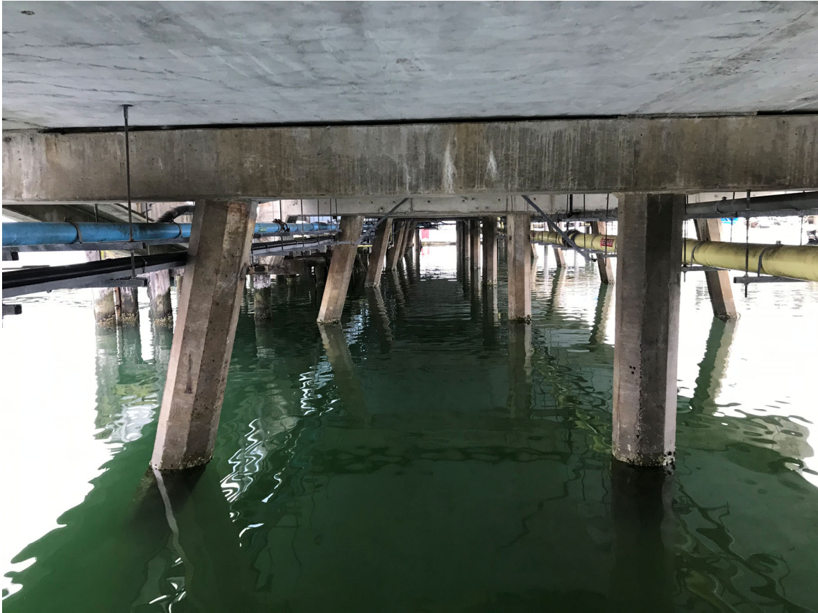
6 – View of support piles, deck, bents and utilities under pier
