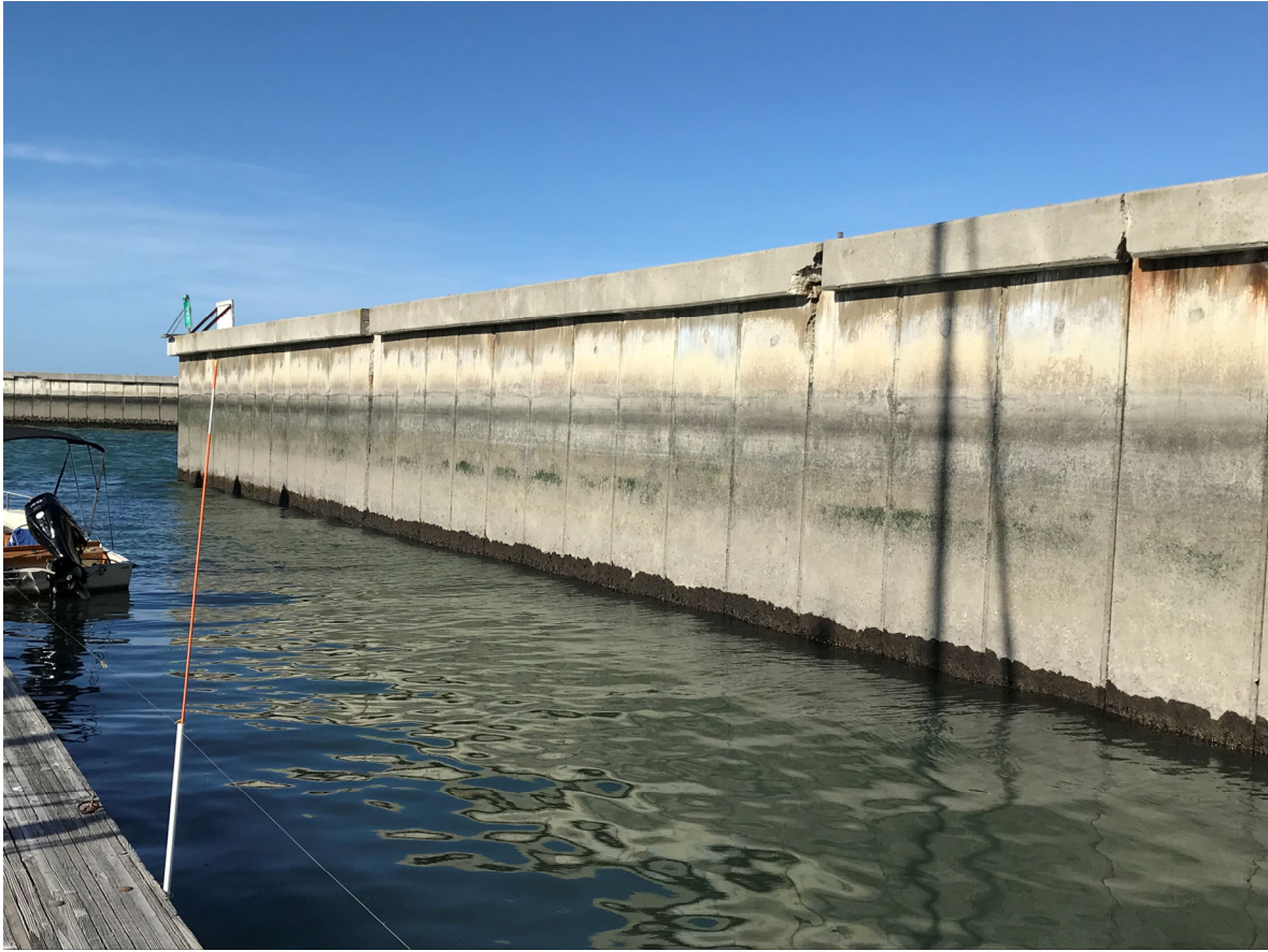
46 – View of seawall
