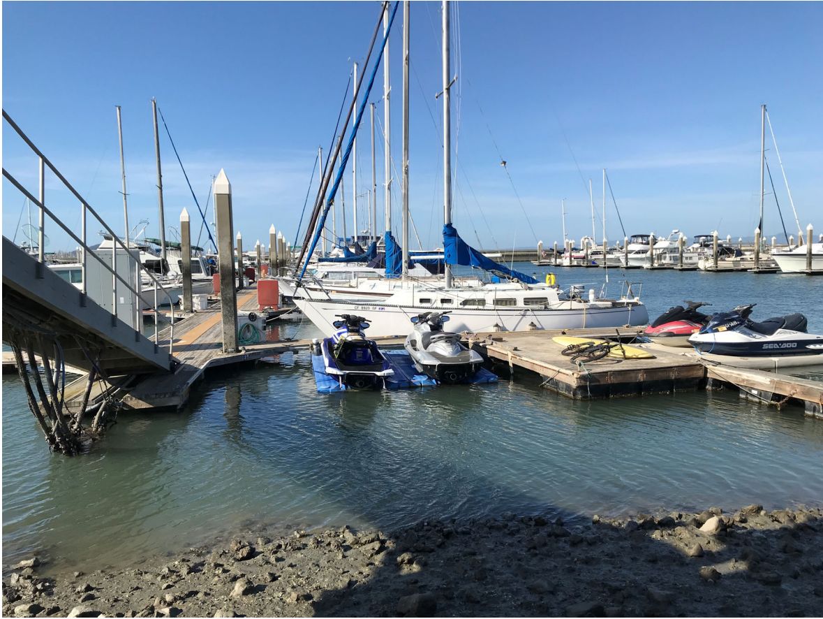
34 – View of East Basin Dock 12
