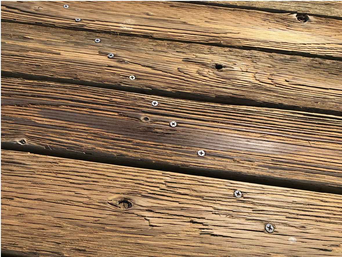
8 – View of stainless steel deck screw on Dock 2
