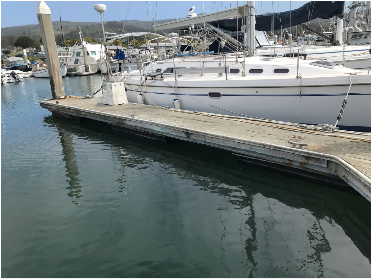
54 – View of typical Dock B finger
