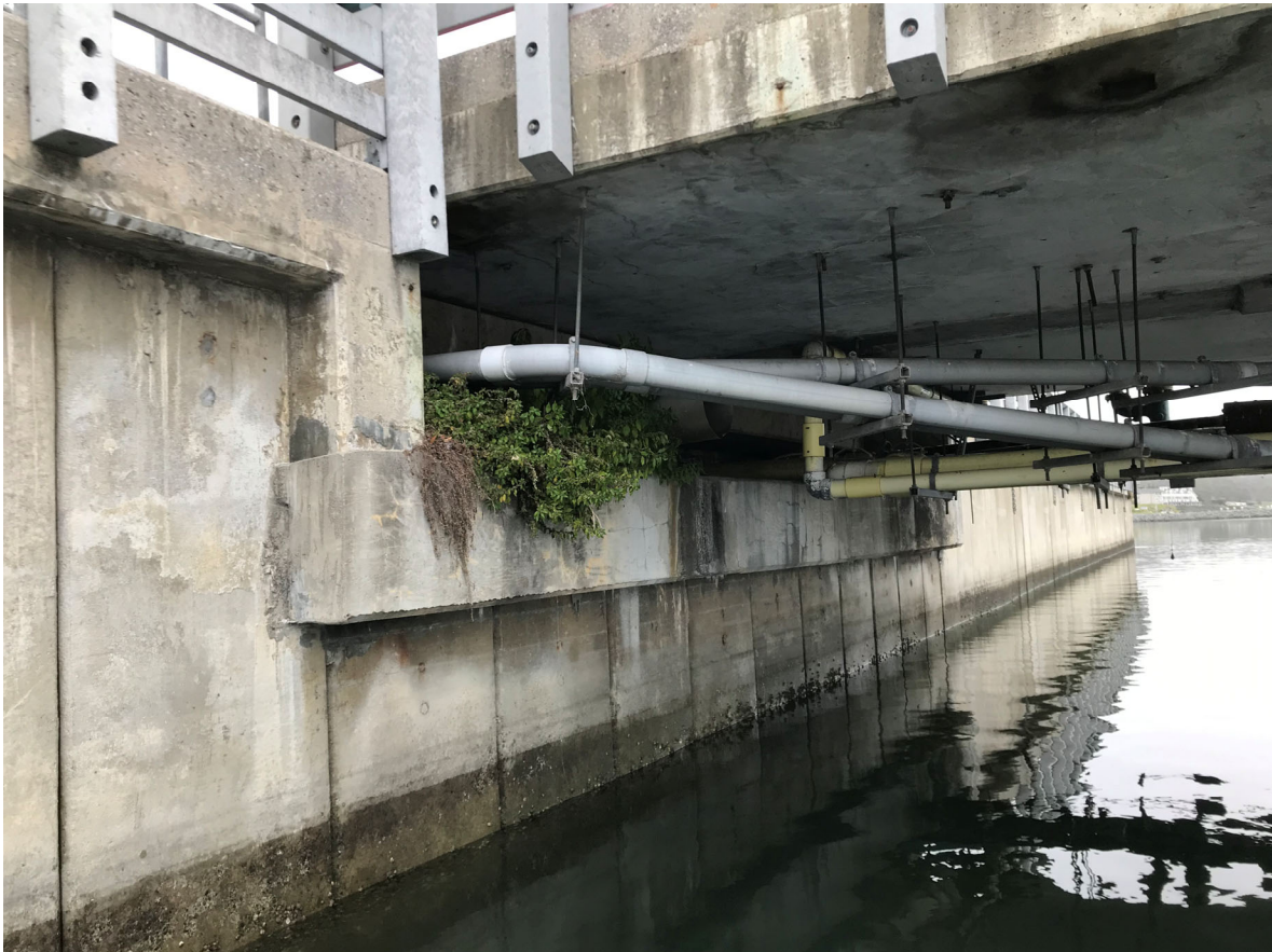
5 – View of utilities under base of pier
