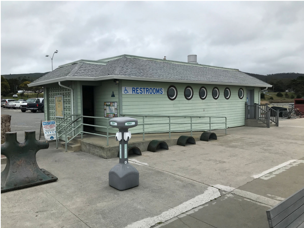
32 – View of Central Restroom exterior and access
