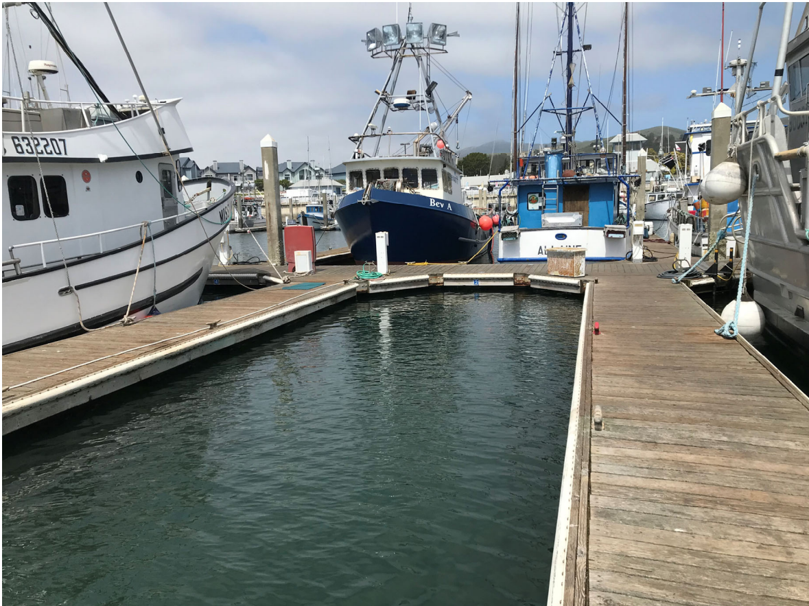
67 – View of Dock H berth
