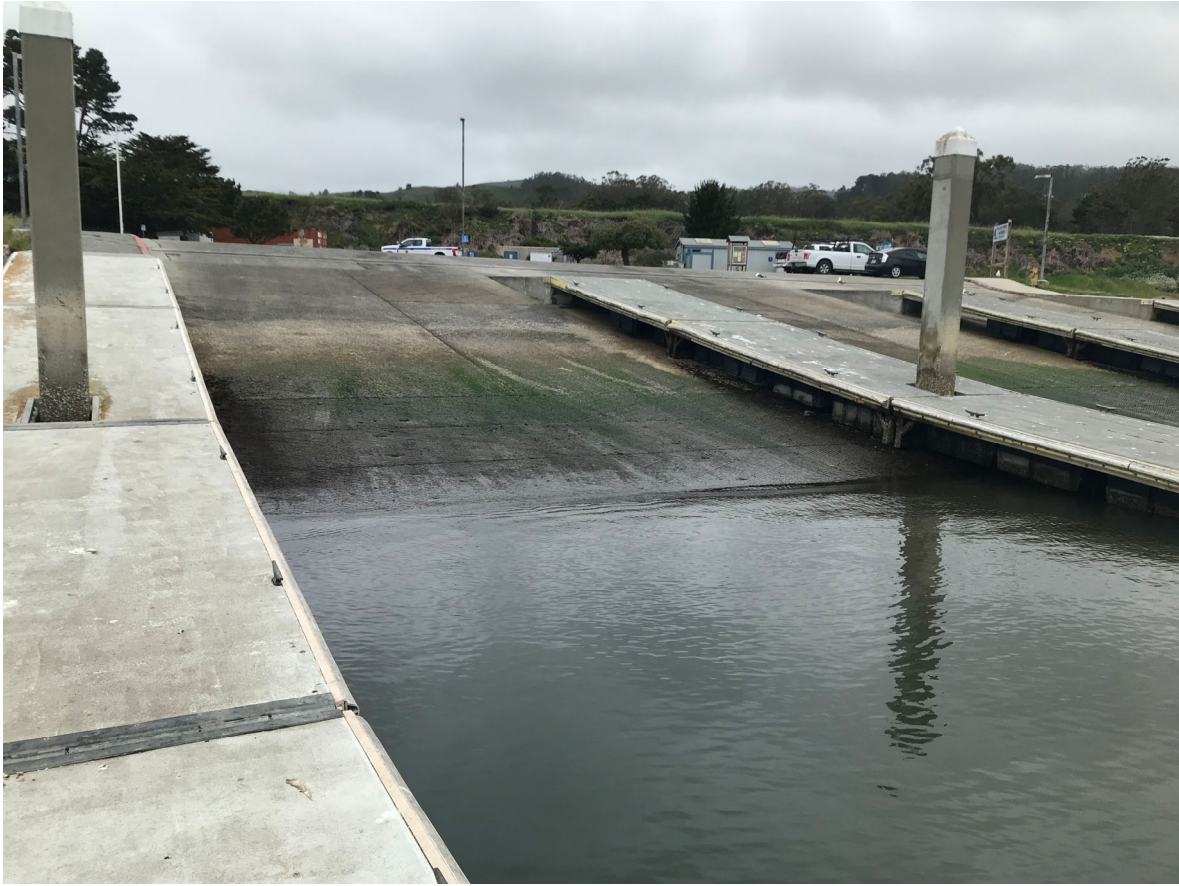
42 – View of boat launch ramp and boarding docks
