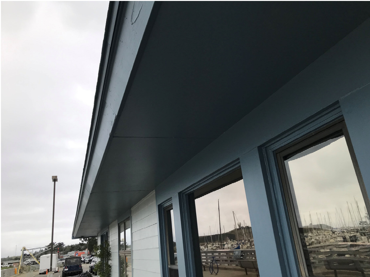
31 – View of Harbor Office Building exterior soffit and added security lighting
