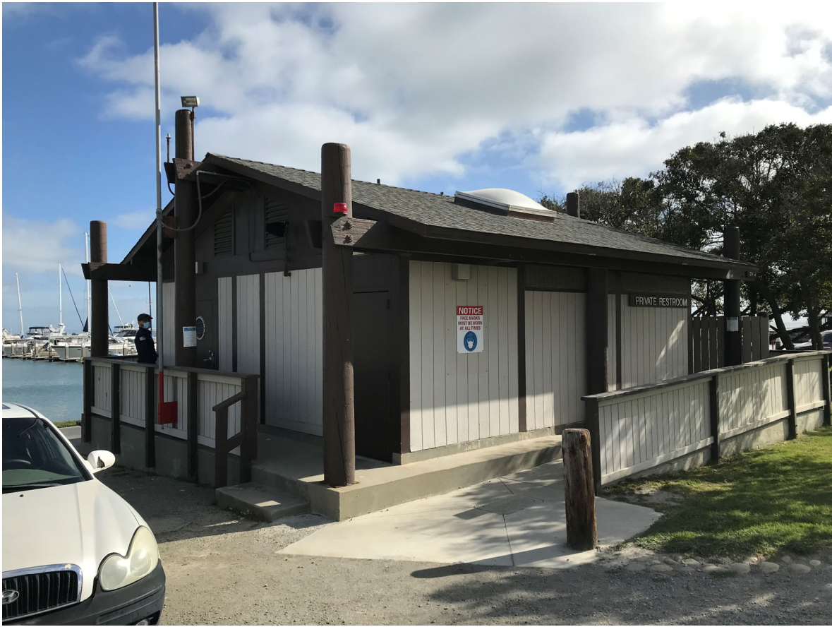
58 – View of East Basin Restroom 2 near Docks 12 and 13
