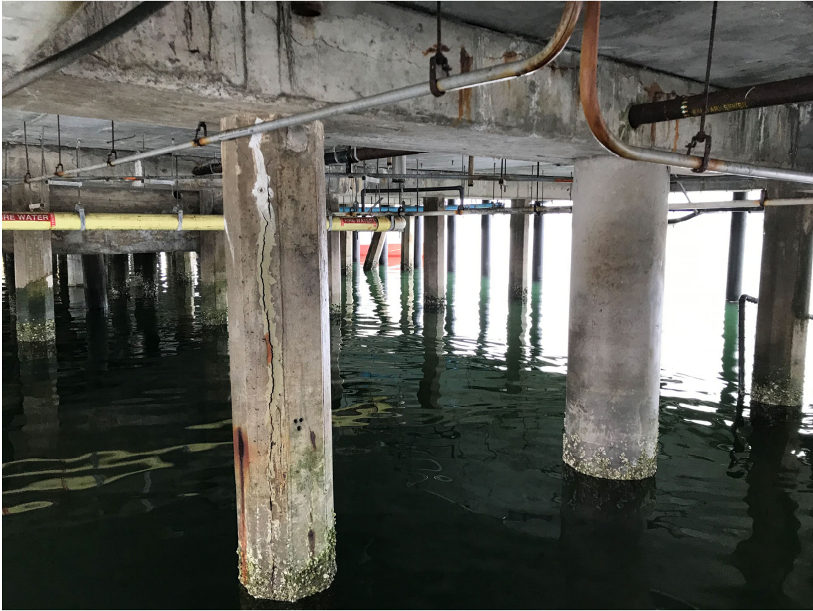
10 – View of support pile and bent at end of pier
