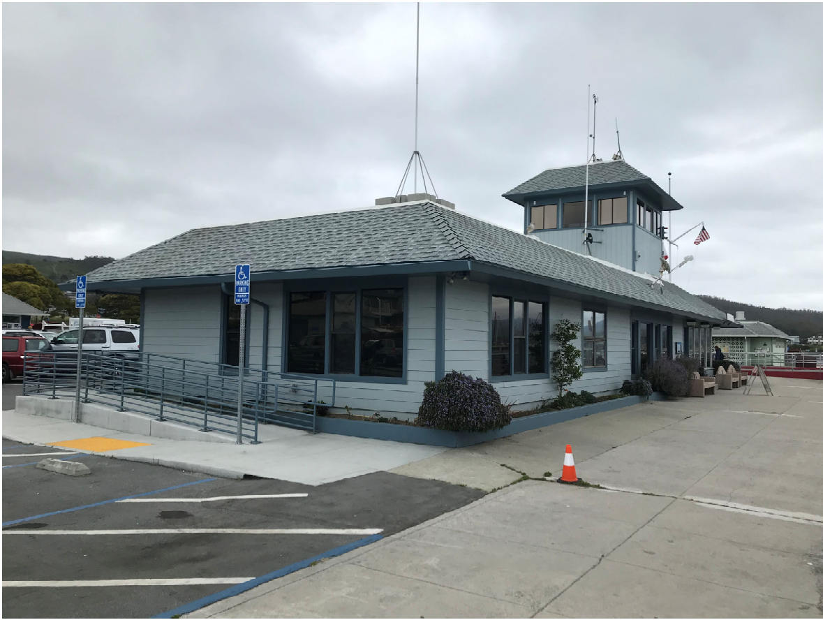
30 – View of Harbor Office Building (recently renovated and ADA improvements added)
