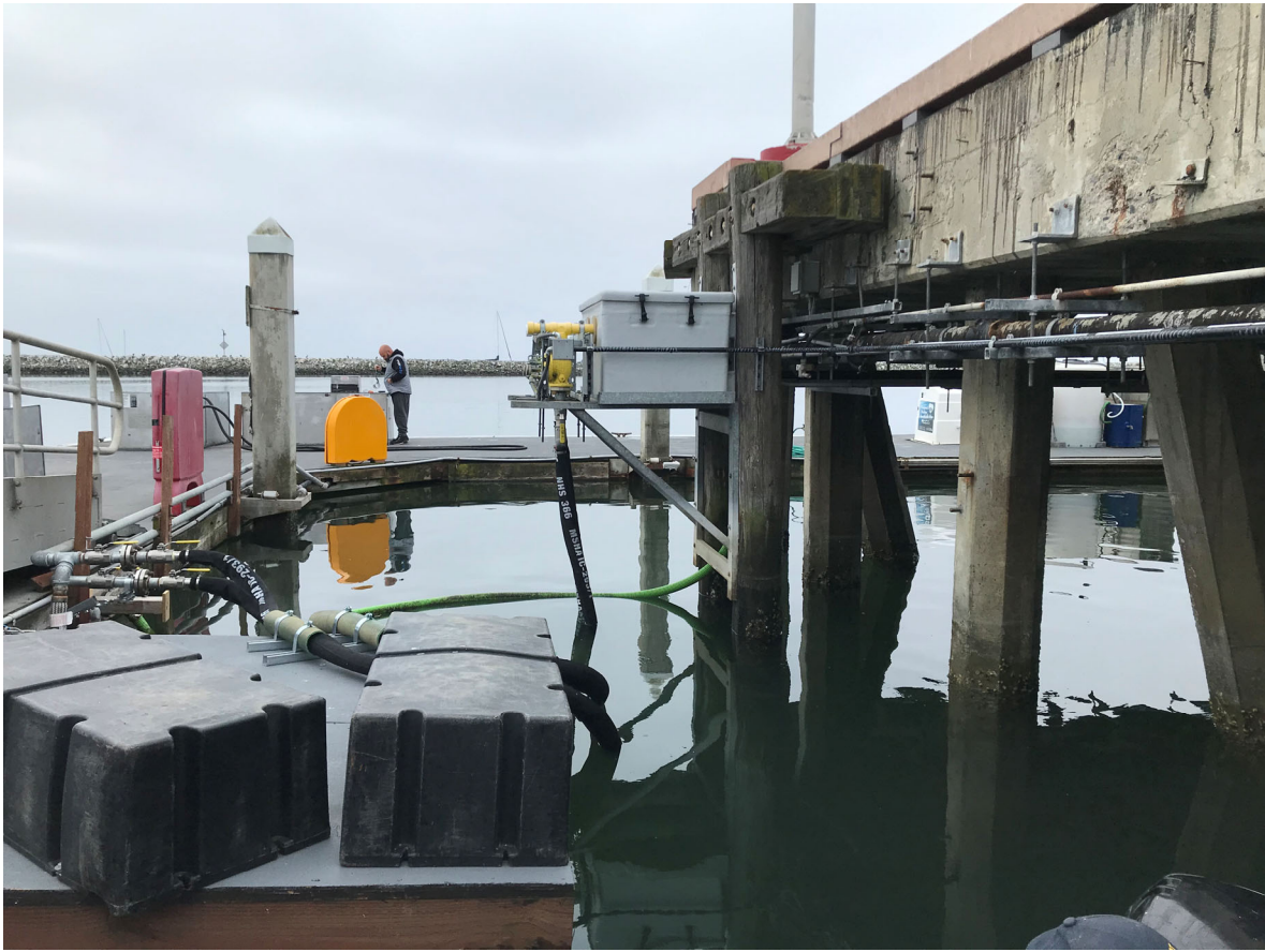
70 – View of Fuel Dock piping from pier to dock
