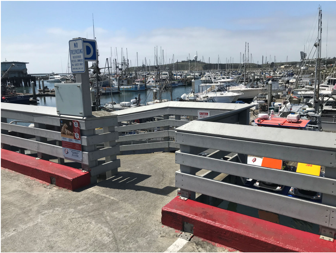
56 – View of access to D Dock from pier
