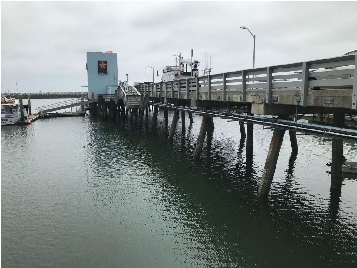
3 – View of east side of Johnson Pier
