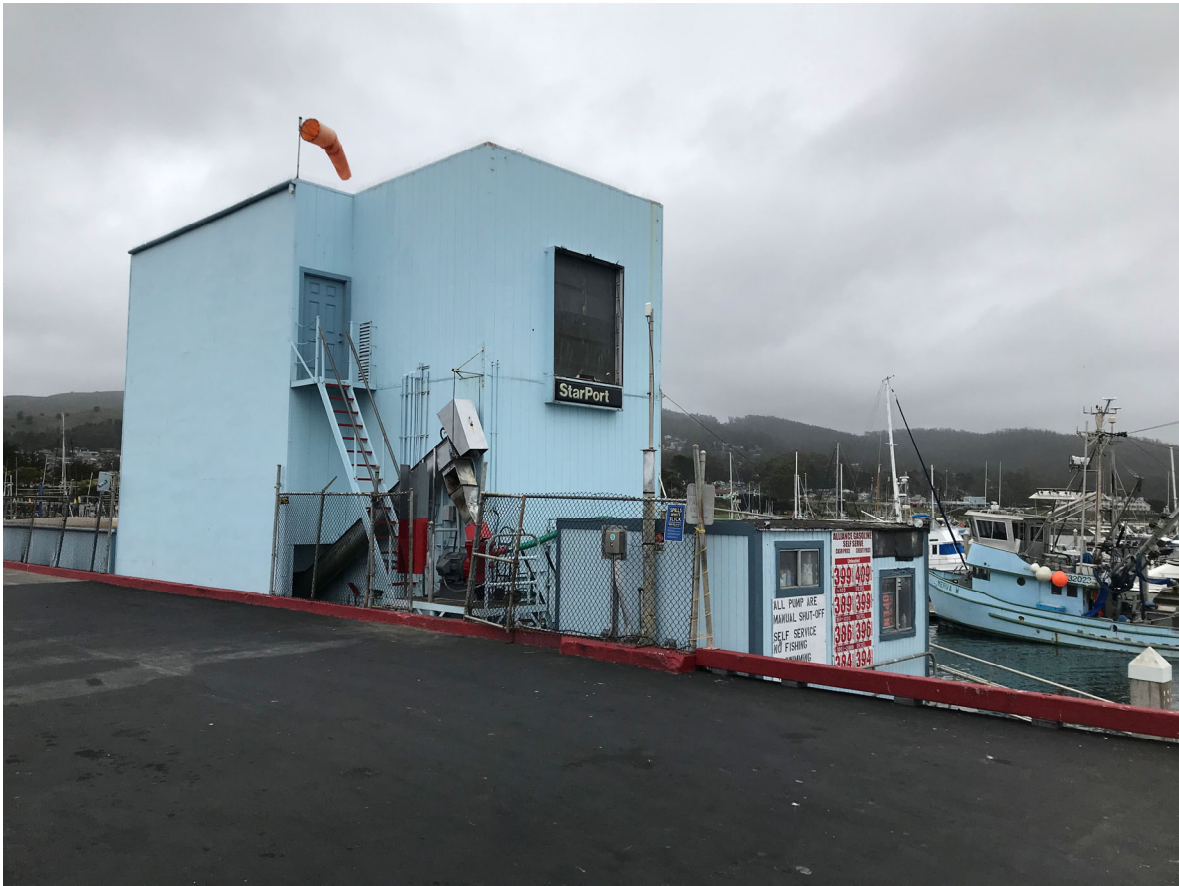
14 – View of Ice House Building and Fuel Dock modular office
