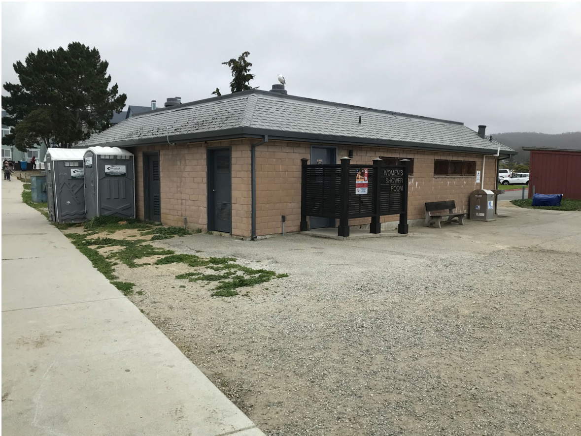
26 – View of West Restroom adjacent to A-C Docks
