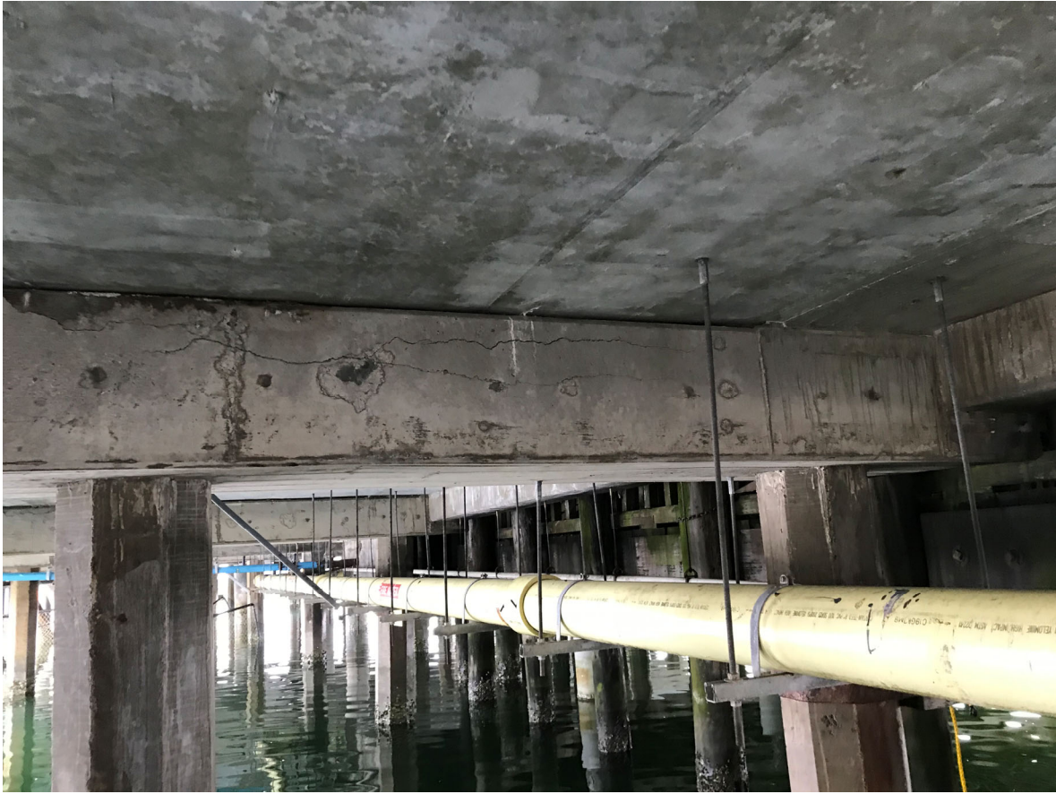
8 – View of support beam and utilities under end of pier
