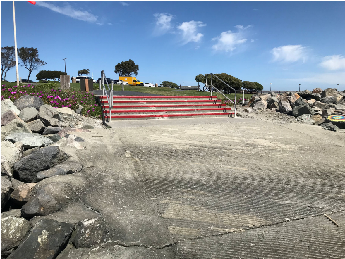
76 – View of Windsurfer launch area
