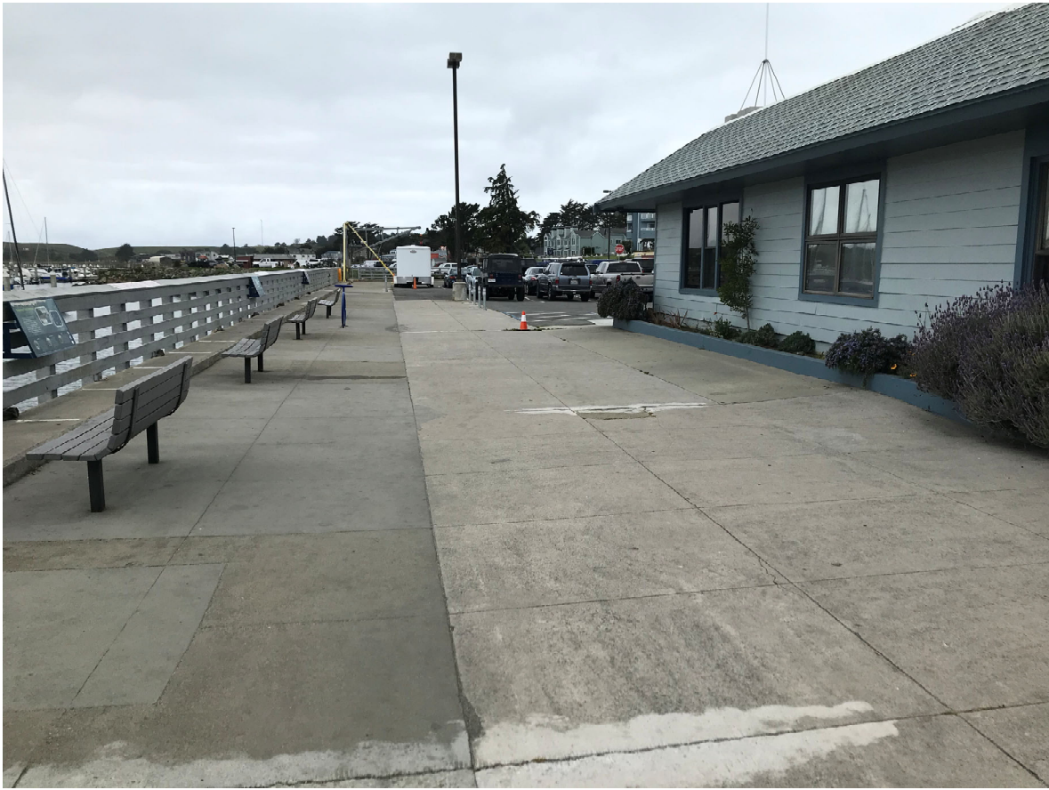
18 – View of promenade in front of Harbor Office Building
