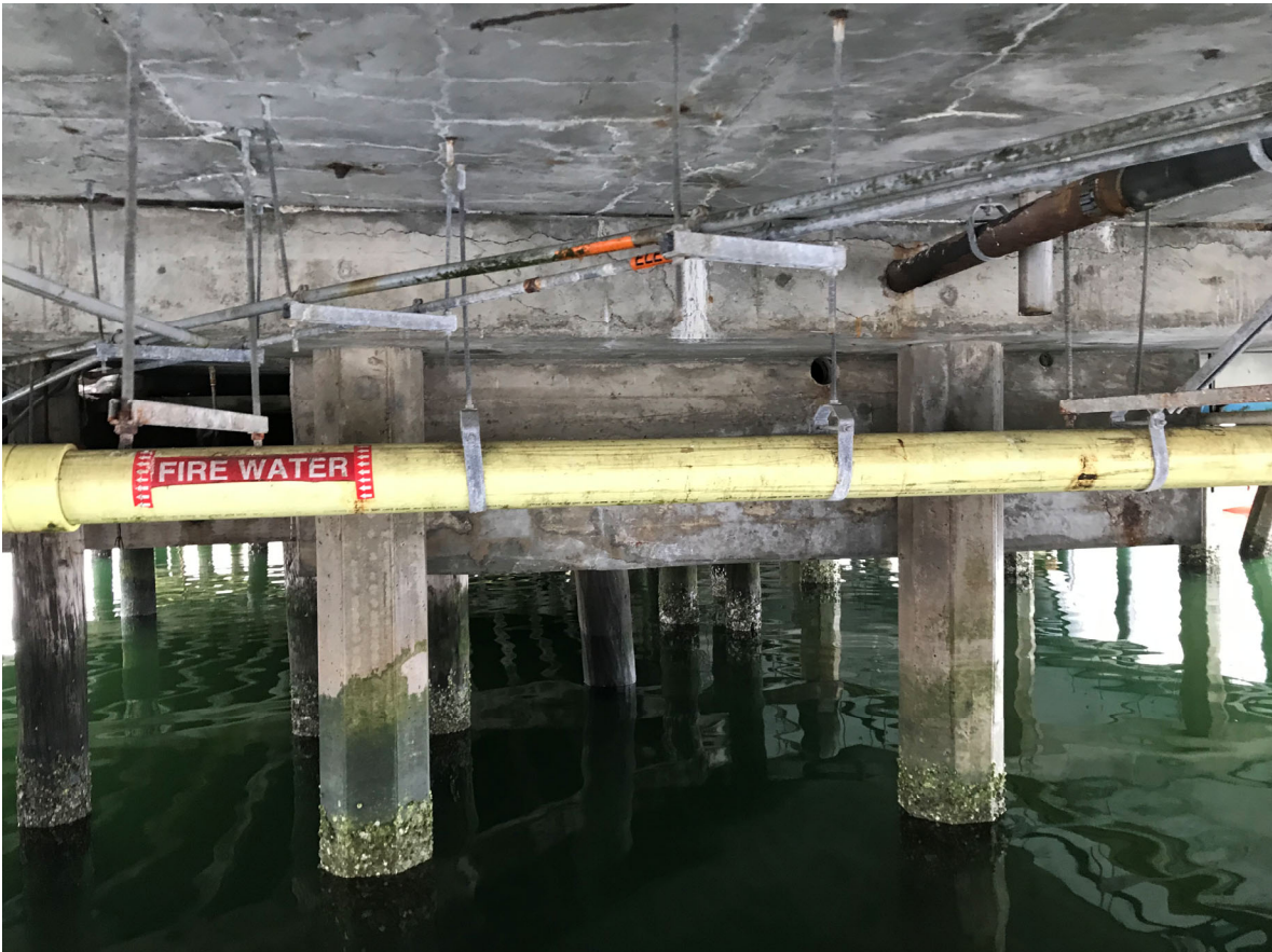
7 – View of support beam and utilities under end of pier
