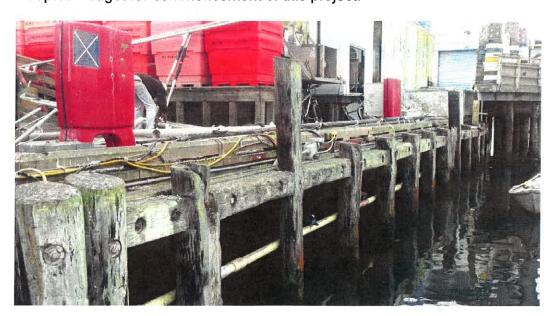
The fender piles in this location are wood, in deteriorated condition and would need to be replaced prior to any use of this area of the pier for off-loading:
