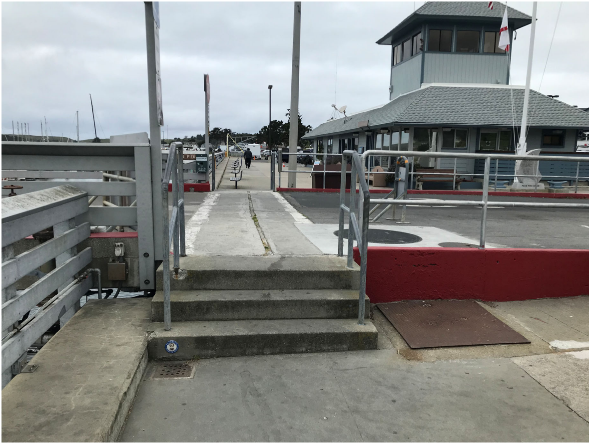
4 – View of 3-step stairs at base of pier
