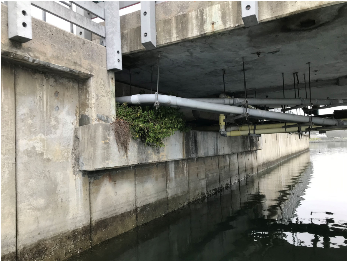
5 – View of utilities under base of pier
