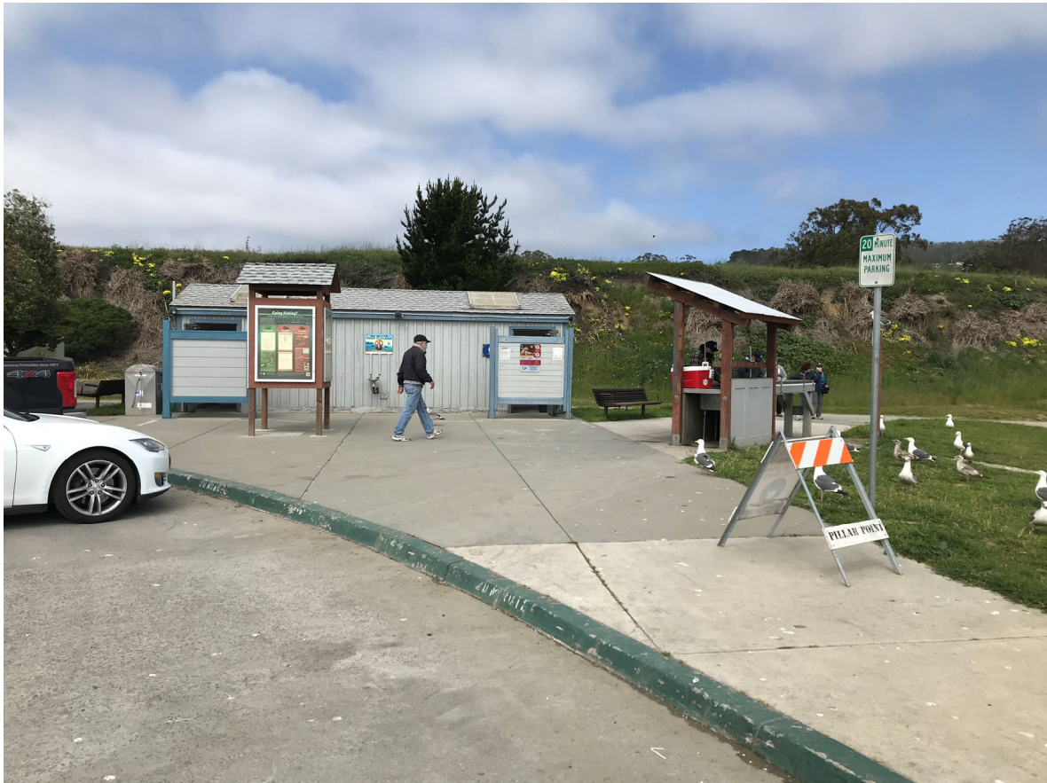
45 – View of East Restroom and fish cleaning station
