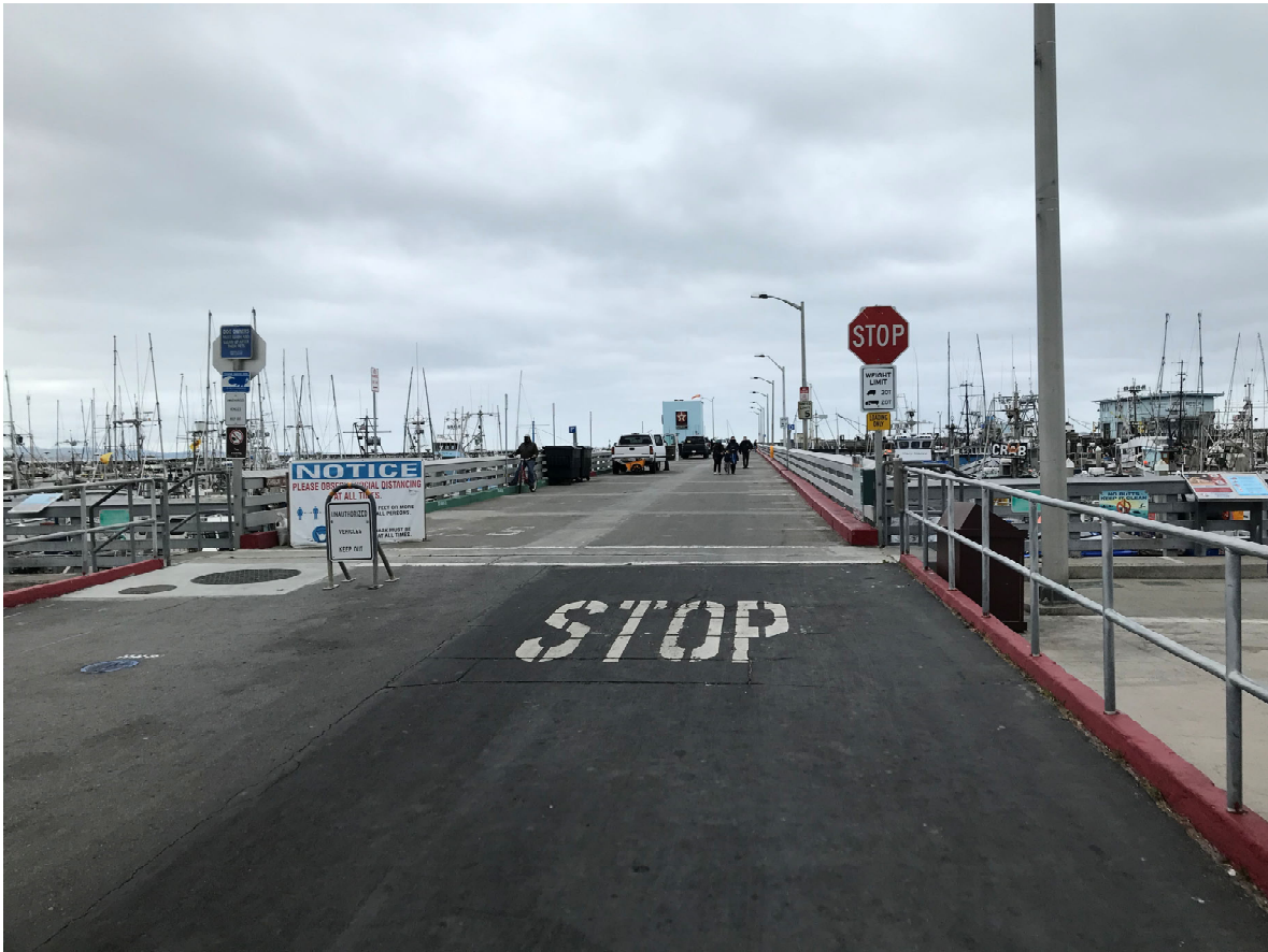
16 – View of pier from landside promenade / access road
