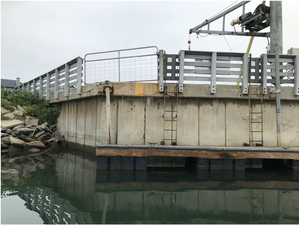
20 – View of west end of sheet pile wall and public hoist
