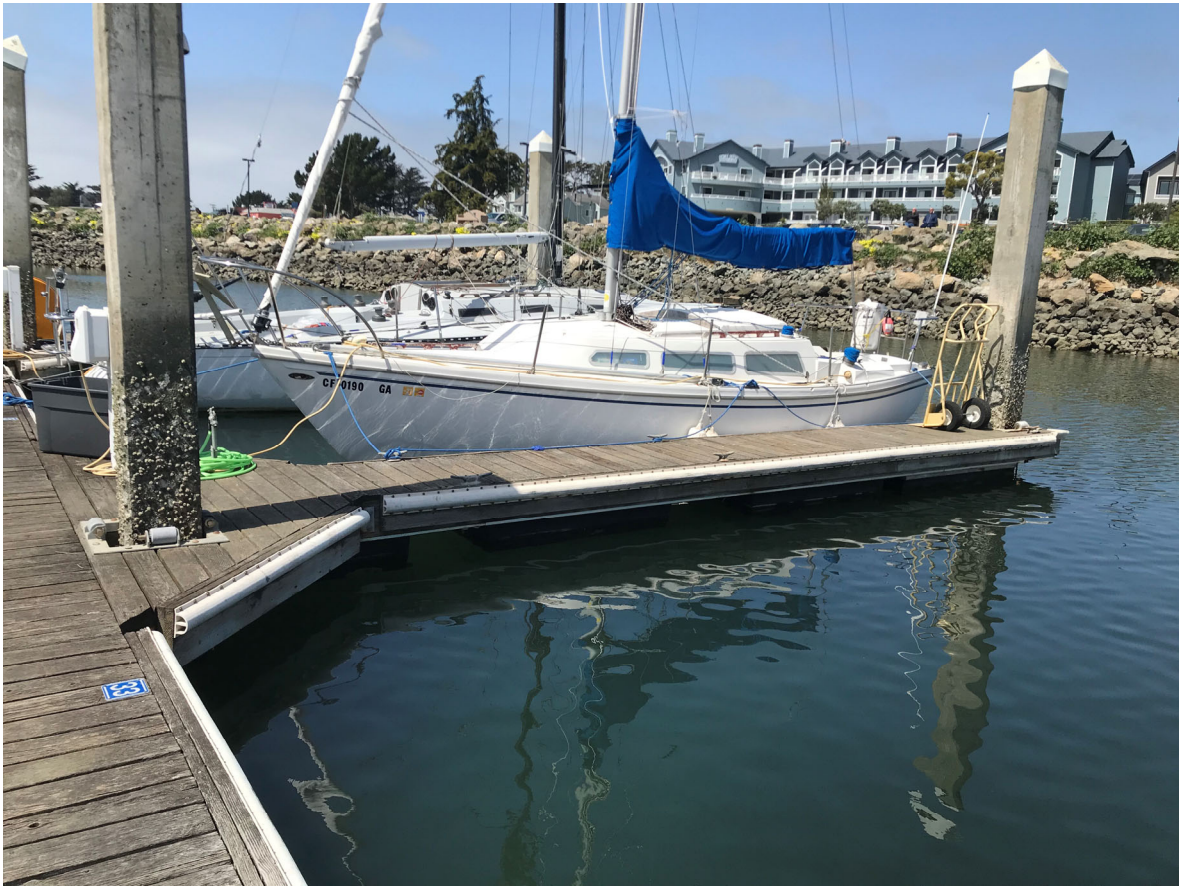
58 – View of typical Dock D finger
