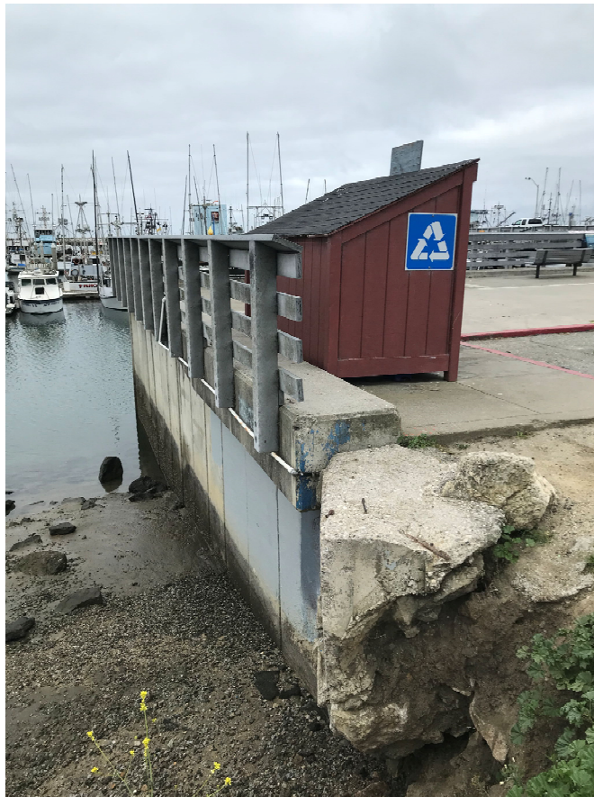
19 – View of promenade and east end of sheet pile wall (with exposed concrete block)
