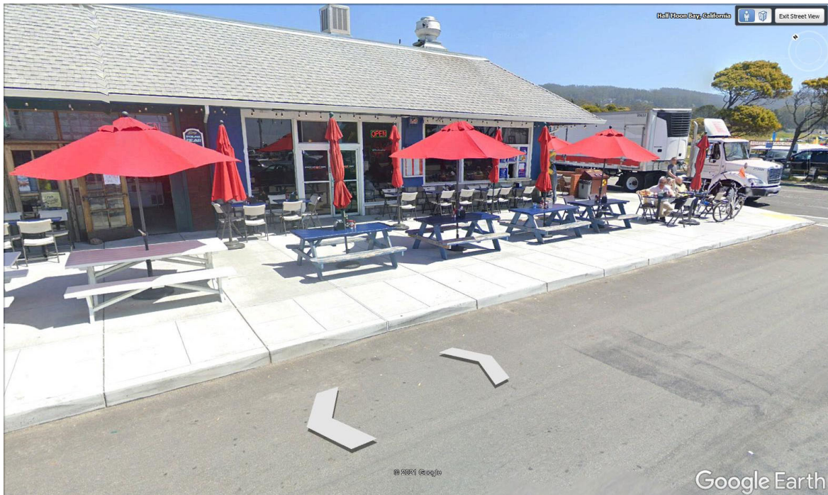
34 – View of Tenant Row Building extended patio seating (Google Earth Pro)
