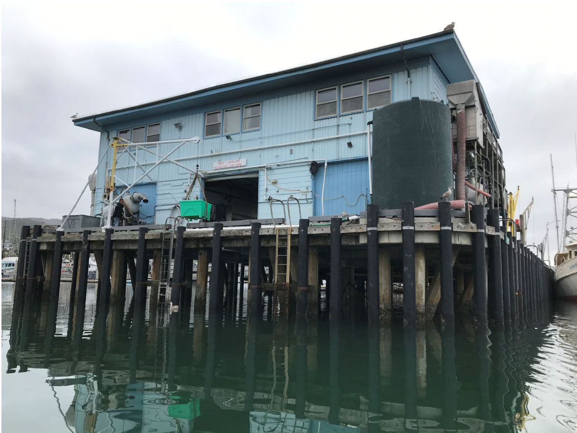
11 – View of Fish Buyer Building at end of pier
