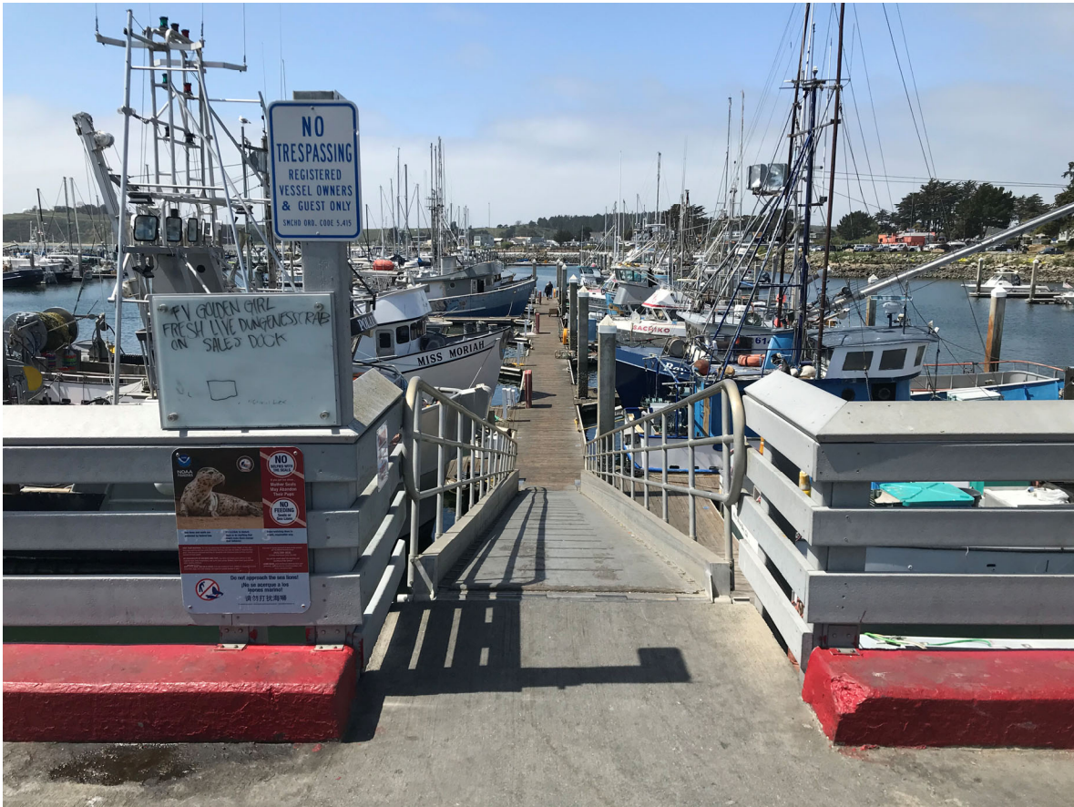
60 – View of entrance to Dock E
