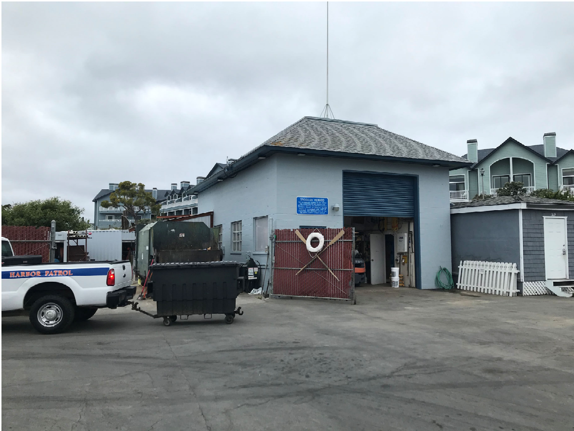
28 – View of Maintenance Building
