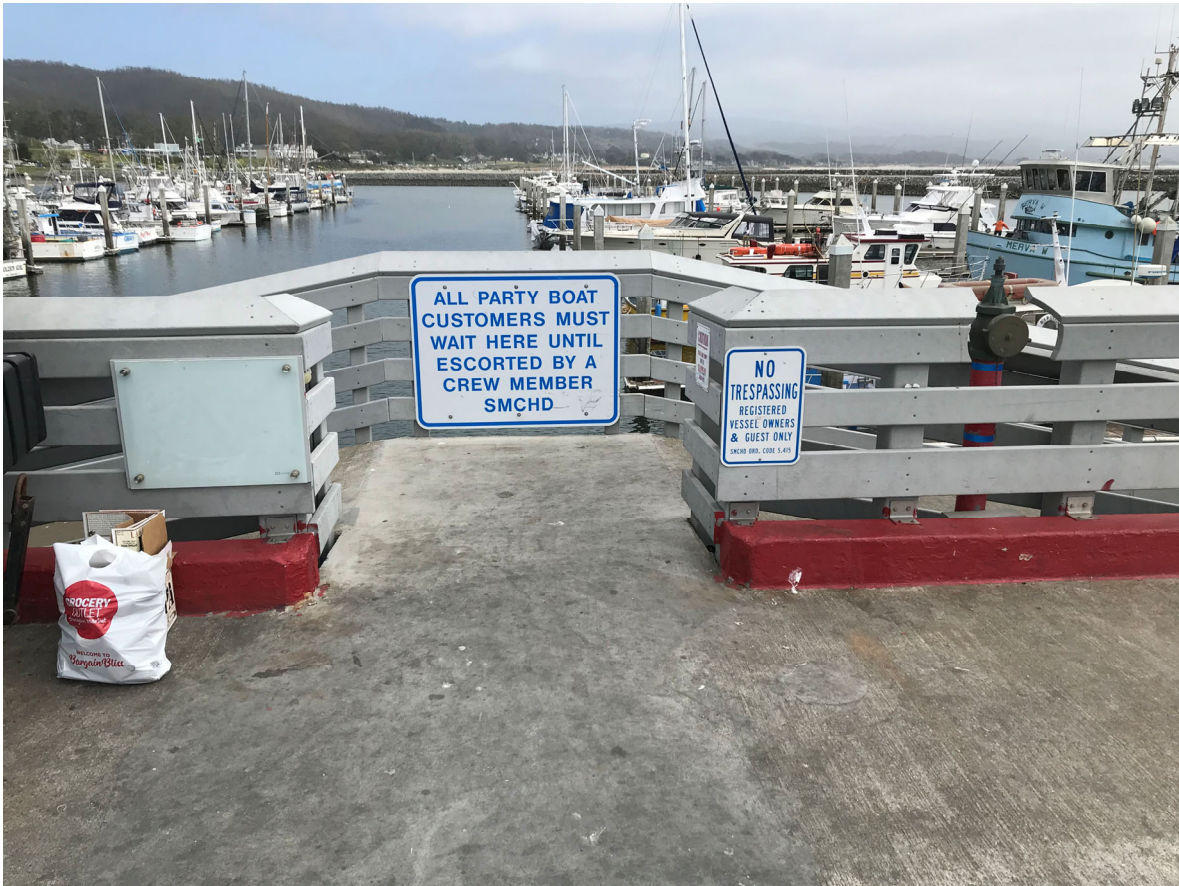
66 – View of entrance to Dock H
