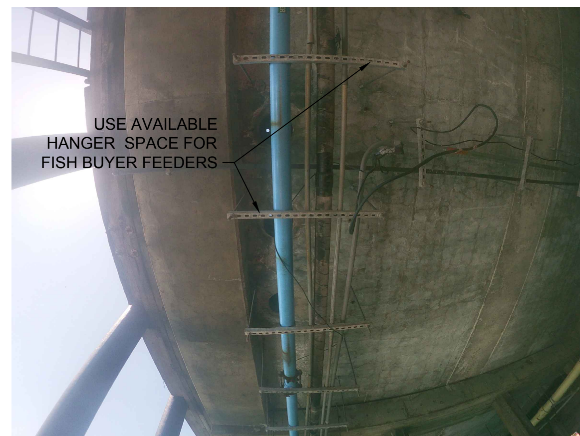
5 EXISTING SOUTH SIDE PIPE HANGERS EP01 SCALE: NTS
