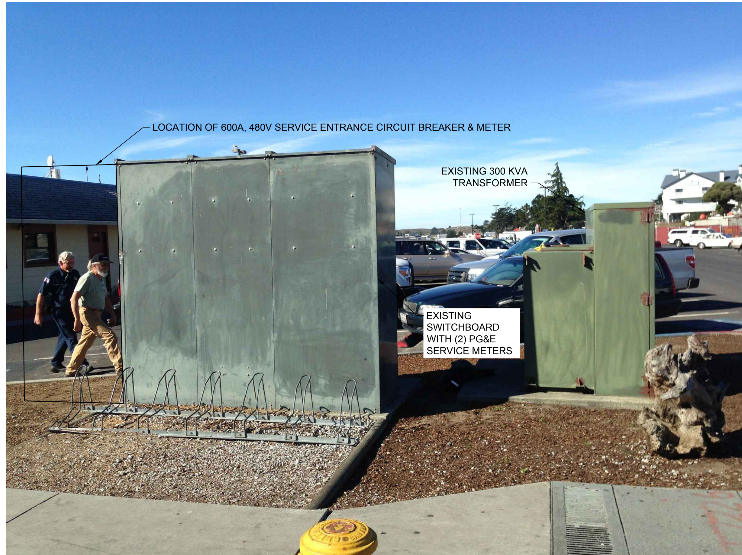
1 EXISTING UTILITY SERVICE AREA EP41 SCALE: NTS
