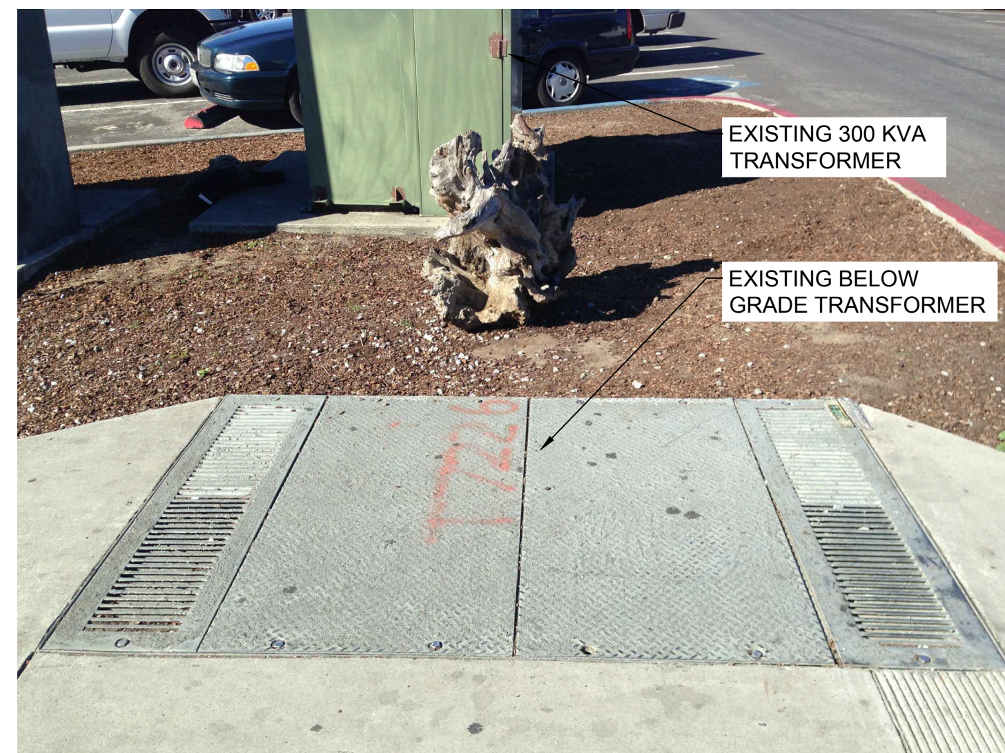
2 EXISTING BELOW GROUND TRANSFORMER EP41 SCALE: NTS
