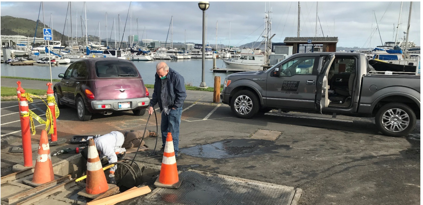
Figure 21. Oyster Point Marina – Electrical Pull Box Being Maintained to Dock 13, 2021
