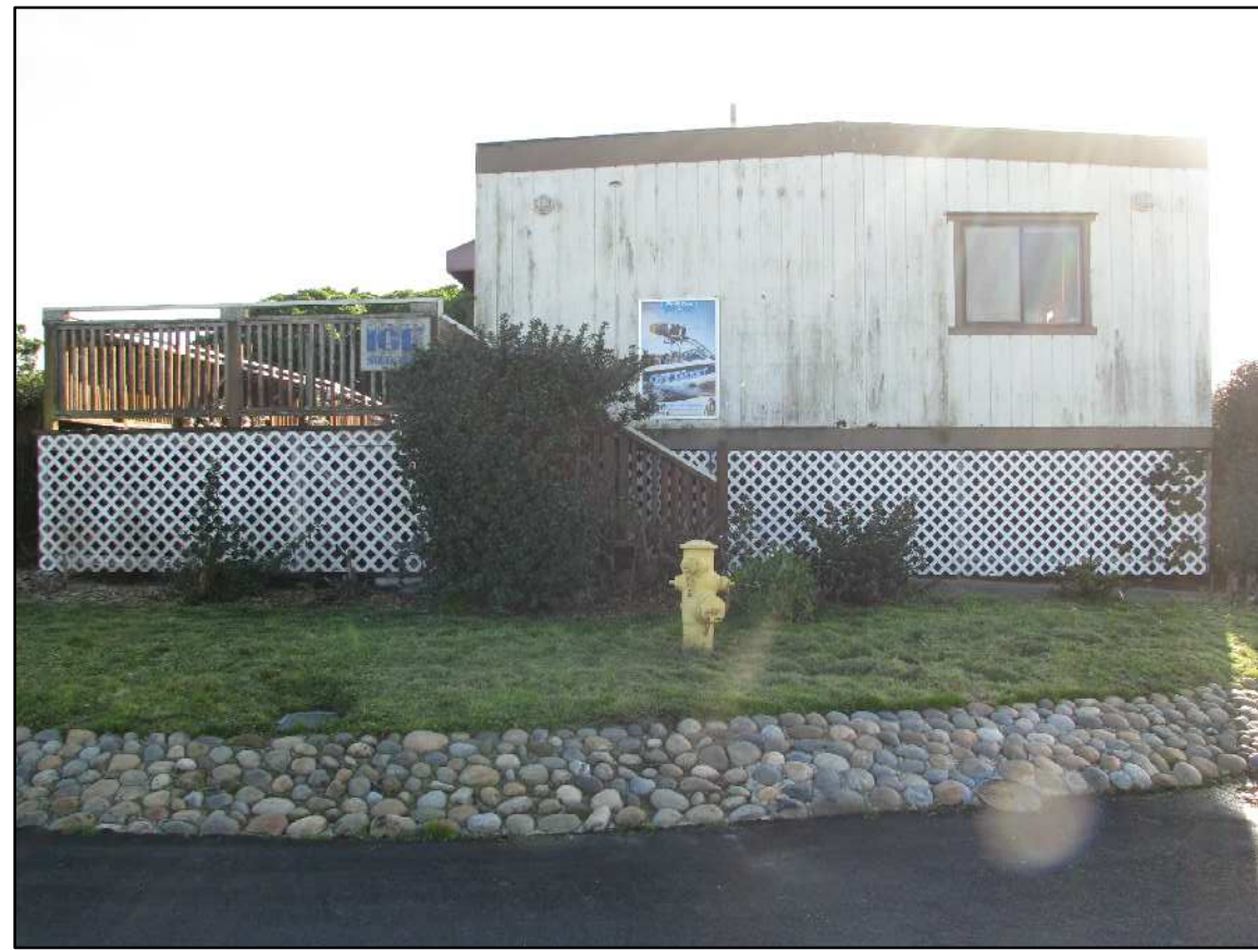
1 NORTH FACE OF BUILDING D-001 - NTS
