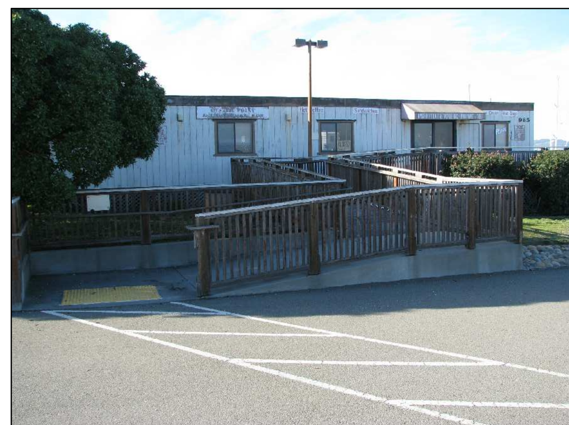
8 EAST FACE OF BUILDING D-001 - NTS
